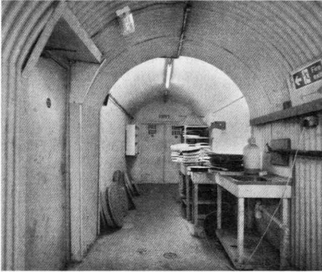
The north parallel corridor leading to one of the two emergency exit tunnels. The entrance tunnels are all lined in brick but many of the tunnels within the shelter are lined with sheets of corrugated metal as seen here.
